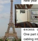
rebuilt this year. The new lighting scheme started operations in June and will remain for 10 years. SDEL IMTEC installed a Centralized Technical Management System to manage in excess of 2500 I/O distributed across 5 S7 PLC's.
