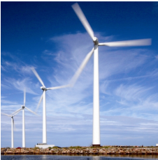
Wind Turbines Synchronization of windmills in a wind park
